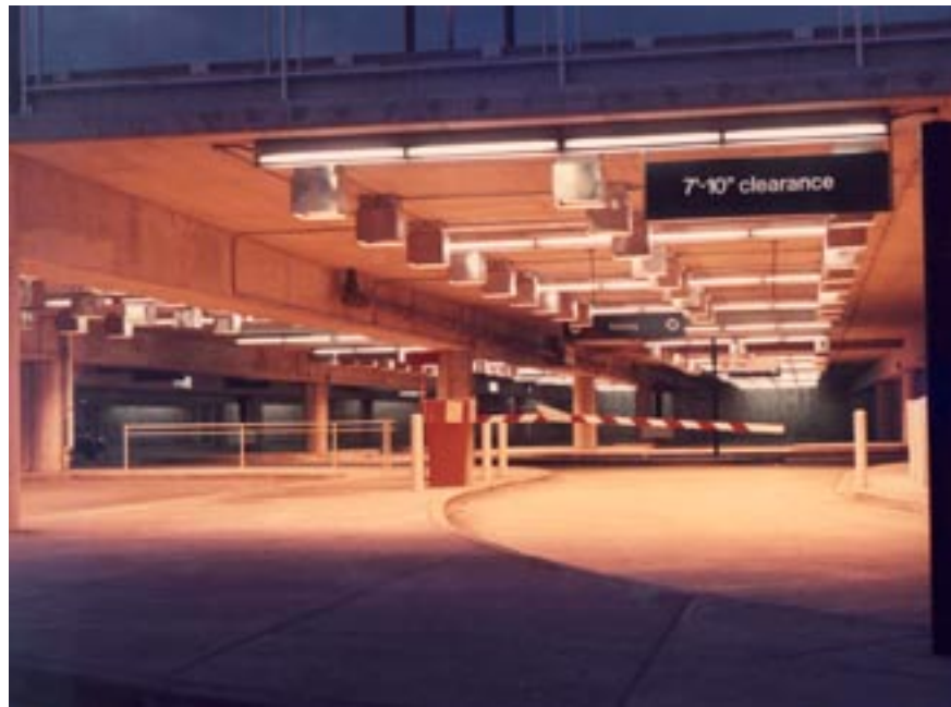
Parking Structure Chicago, IL
