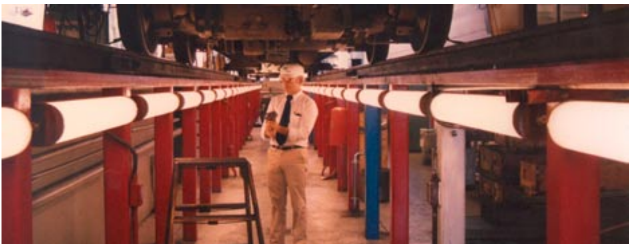
Rapid transit service pit area San Francisco, CA
