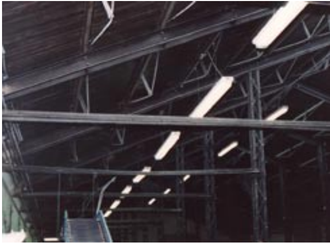
Agricultural processing facility Croswell, MI
